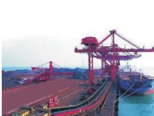
皮带机 Belt conveyer
